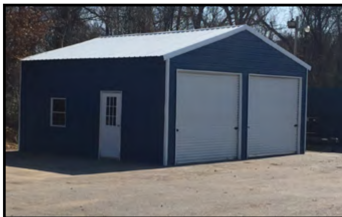
Vertical Garage (Extra Frame work to allow metal to be installed vertical)
